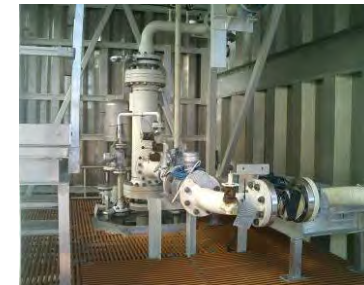
InLine DeSander First application at Statoil Heidrun
